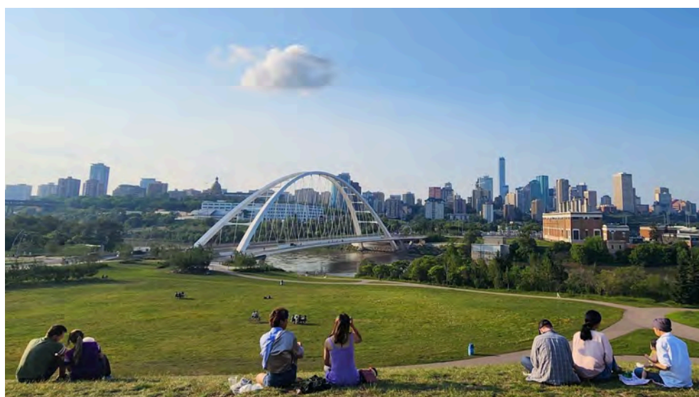
Hilltop view of the Walterdale Bridge and Edmonton's downtown skyline.
