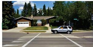
A crosswalk which is constructed higher than the roadway surface.
