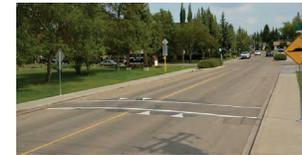
Speed humps are a raised section of the road. They are similar to raised crosswalks but are shorter in length and not placed at crossings.
