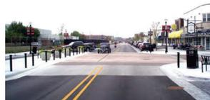
An intersection that is constructed higher than the surrounding roadway surfaces.
