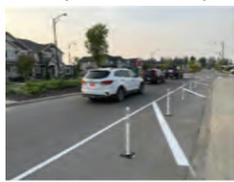
Photo of an Pavement Marking and Reflective Posts on Desrochers Dr. & Desrochers Blvd., as part of the St. Thomas Aquinas School Project.
