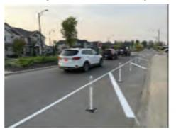
Photo of an Pavement Marking and Reflective Posts on Desrochers Dr. & Desrochers Blvd., as part of the St. Thomas Aquinas School Project.
