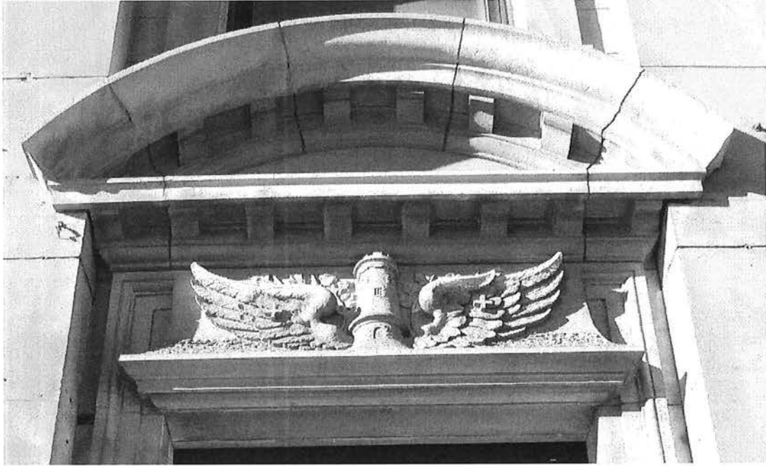
Bas Relief "Winged Lighthouse" and Arched Pediment Above Main Entrance
