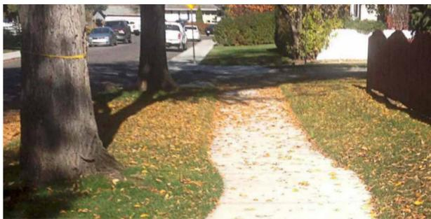
Extra deep cuts and rebar are added to the sidewalk to control where the sidewalk will crack and to keep the sidewalk intact as the tree's roots grow.
