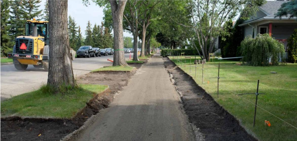
Forms are set in order to pour new concrete for the sidewalk.
