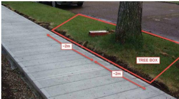
An area around each tree is maintained during construction to protect it and its roots.
