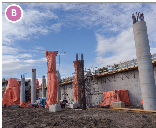
Area 7 - Anthony Henday Drive Bridge Columns & Piles
