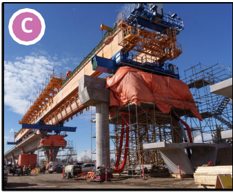
Area 6 - Misericordia Station Elevated Guideway Construction
