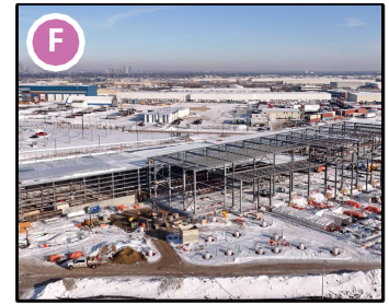
Area 9 - Gerry Wright OMF Construction
