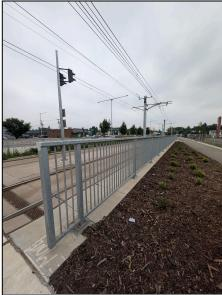
The fencing in the photos above is by the LRT tracks and was installed for safety reasons. This fencing is permanent and part of the design of the Valley Line Southeast.
