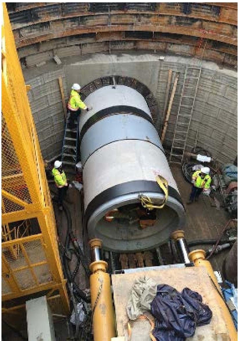
Figure 4. SESS SA1a – Pipe Jacking station in the working shaft at MH 103
