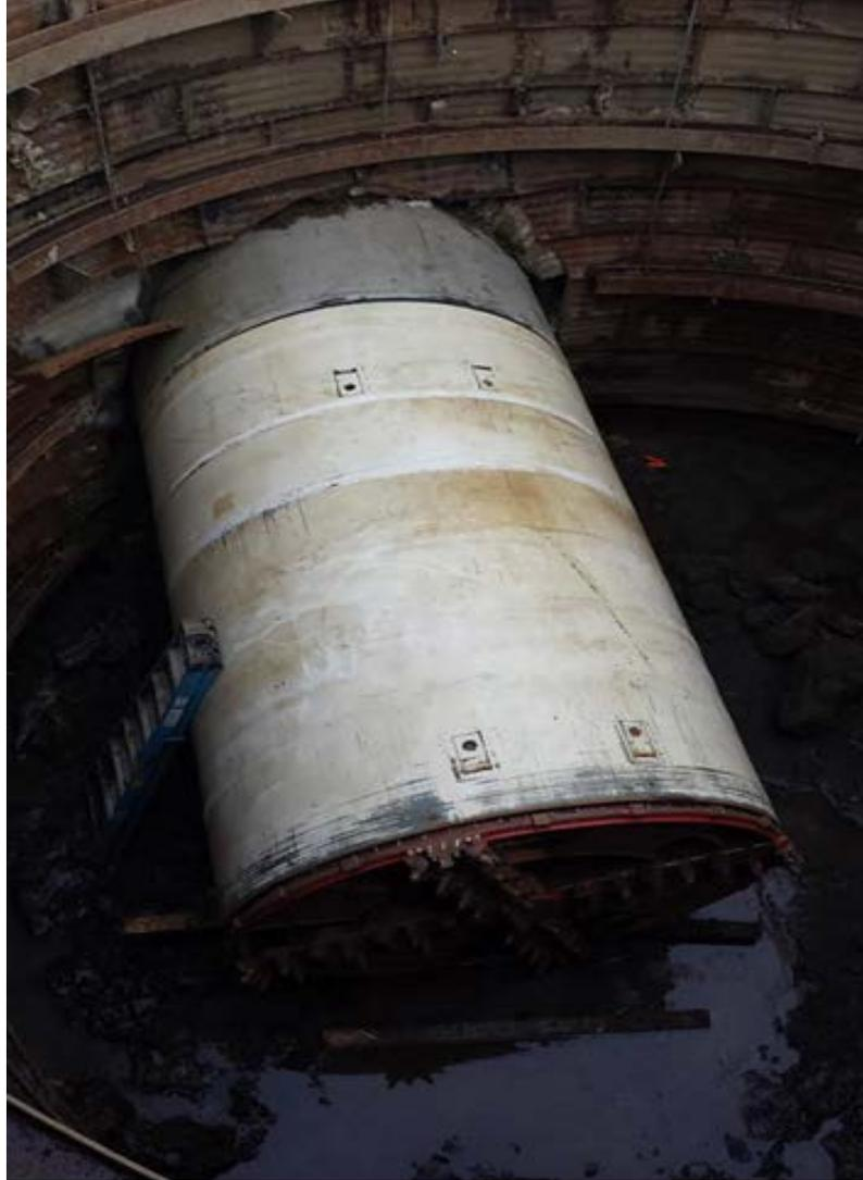
Figure 3. SESS SA1a- TBM head breaking through the receiving shaft at MH 102
