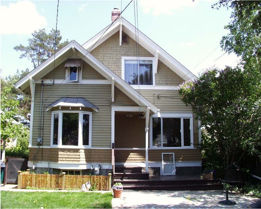
Photo #3 – Rear-West Elevation
