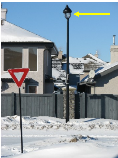
Figure 1: Leaning light fixture
