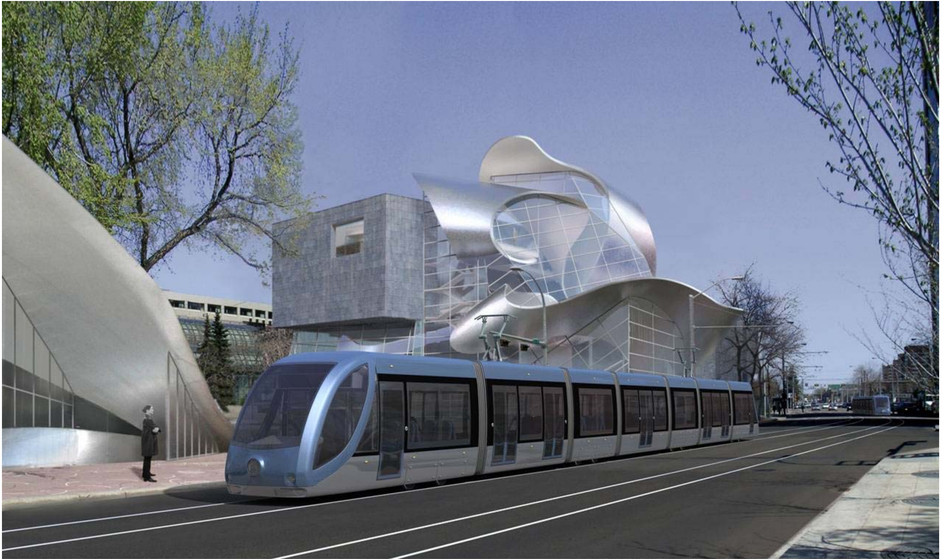
The new Art Gallery of Alberta, opening early 2010. Daytime rendering. Design by Randall Stout, FAIA, RSA, President, Randall Stout Architects Inc.
