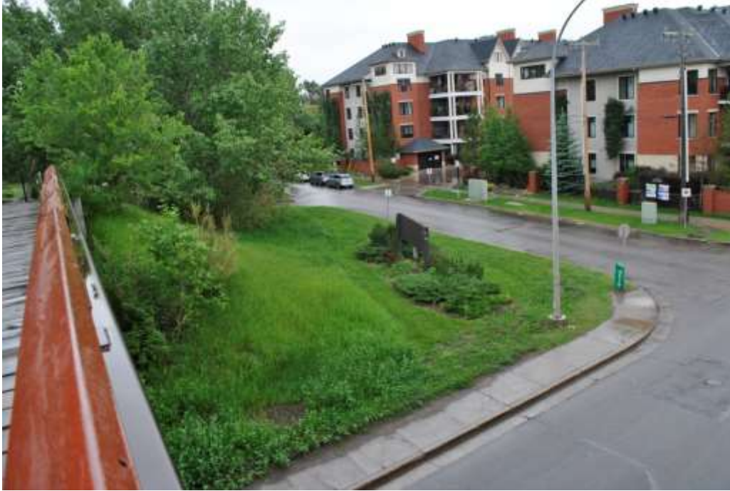
Plate 6.1: Bridge abutment fill in the parcel to be added to the Project Area, looking northeast (June 2014).
