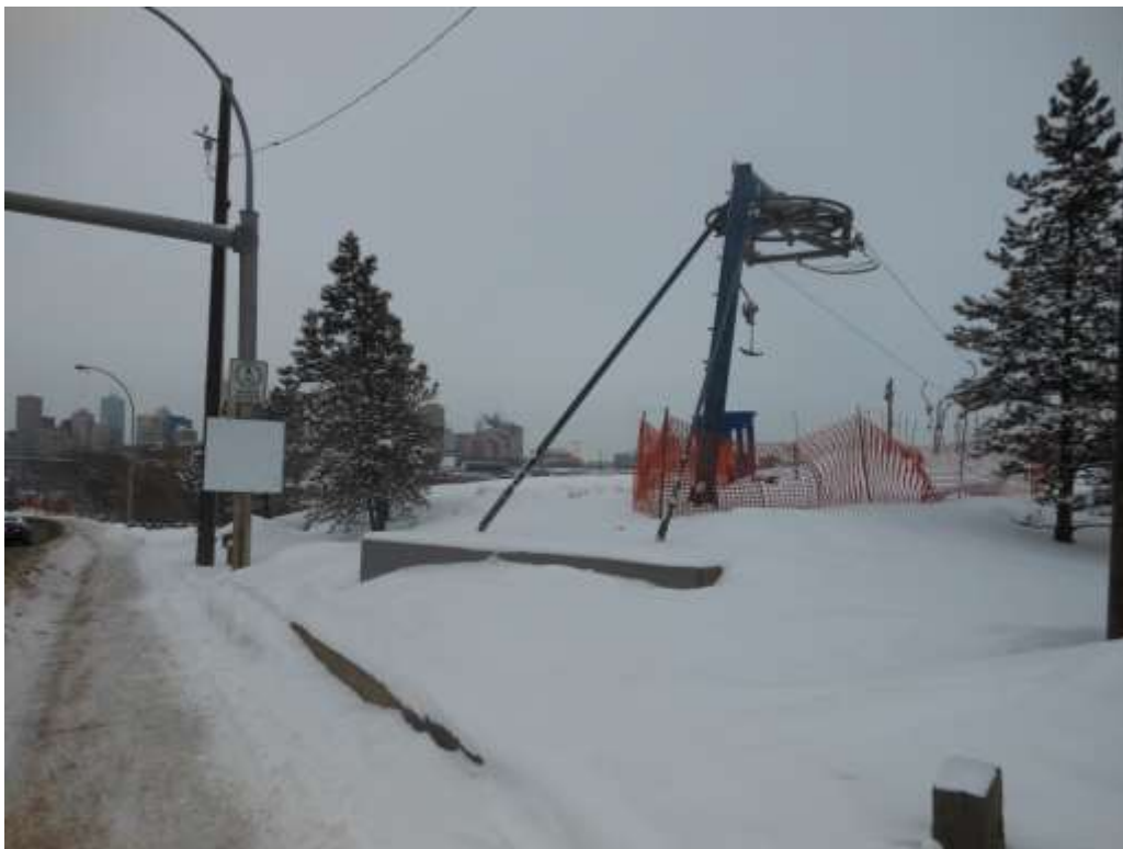
Plate 8.4. The existing T-bar terminus is clearly visible from Connors Road, dominating views at the crest of the hill, looking northwest (Jan. 2015).
