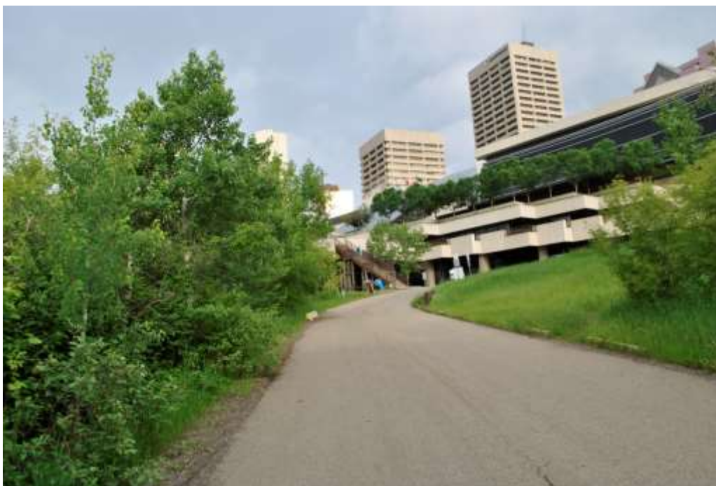
Plate 2.1. Segment of proposed Louise McKinney Riverfront Park Construction Access Road using existing maintenance road, looking northeast.
