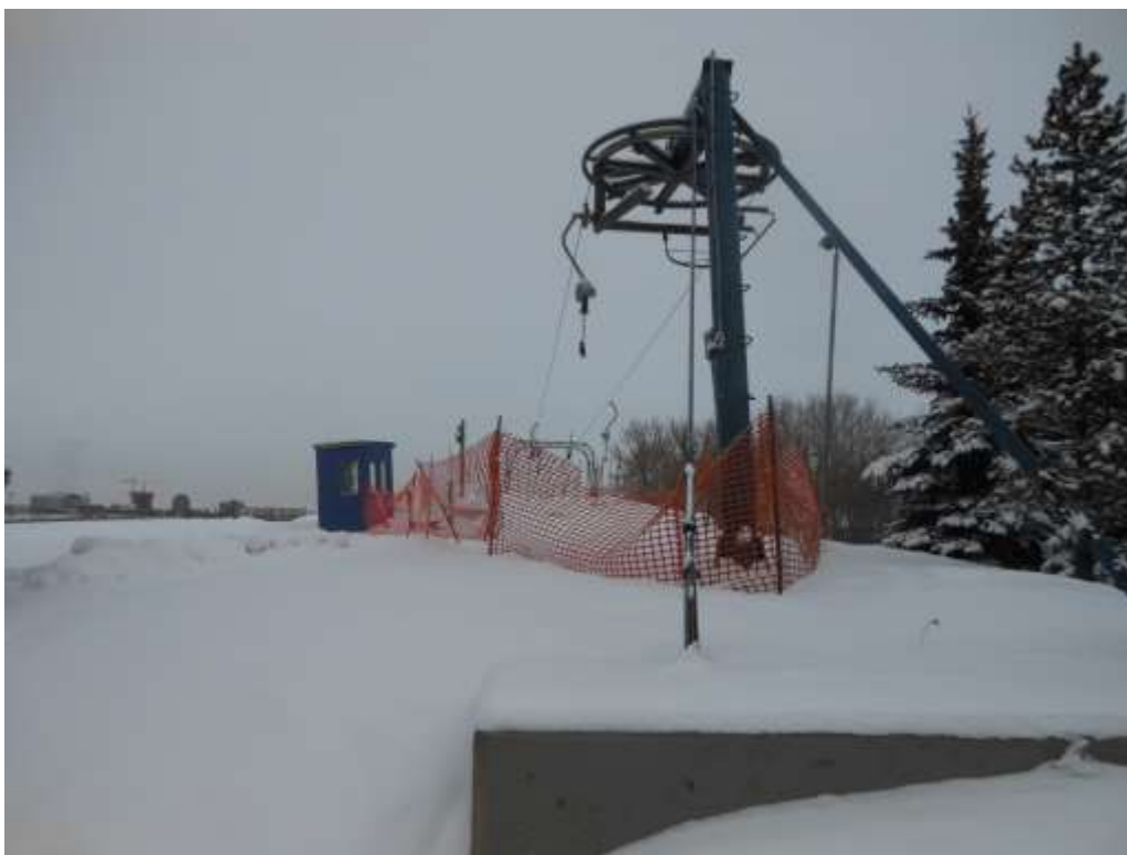
Plate 2.6. Edmonton Ski Club return terminal bullwheel (foreground), operator shack (middle ground) and last tower (background) for the T-bar run, looking northwest (Jan. 2015)
