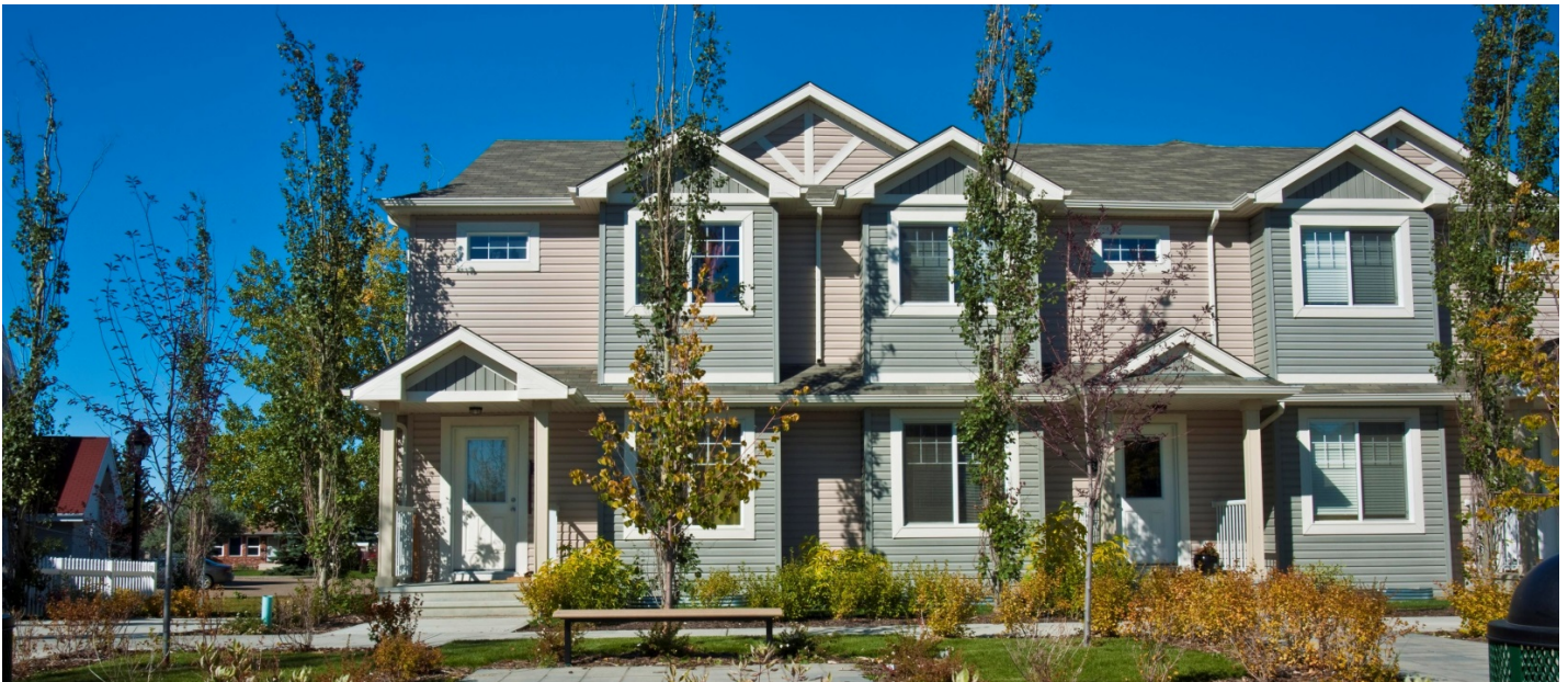
First Place homes on a pilot surplus school site in Greenview sold out immediately
