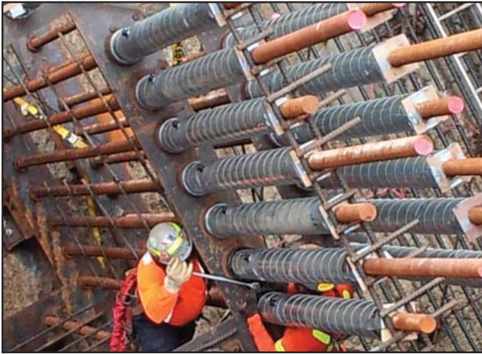
Crew member working on anchor rods.
