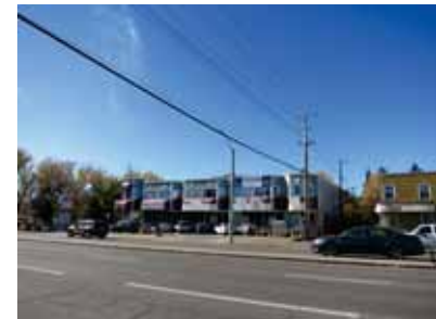
Removal of Overhead Powerlines
