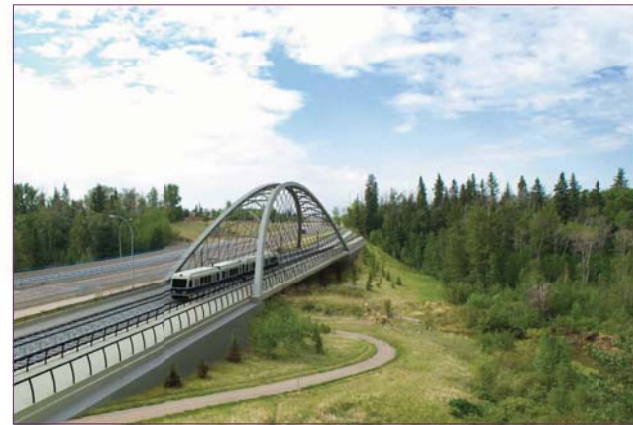
Suspended Arch Bridge
