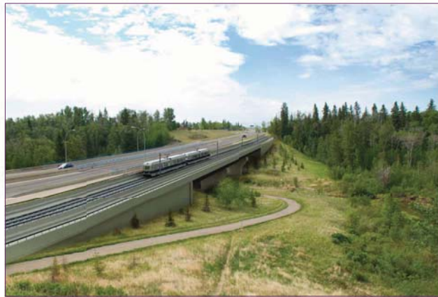
3 Span Girder Bridge
