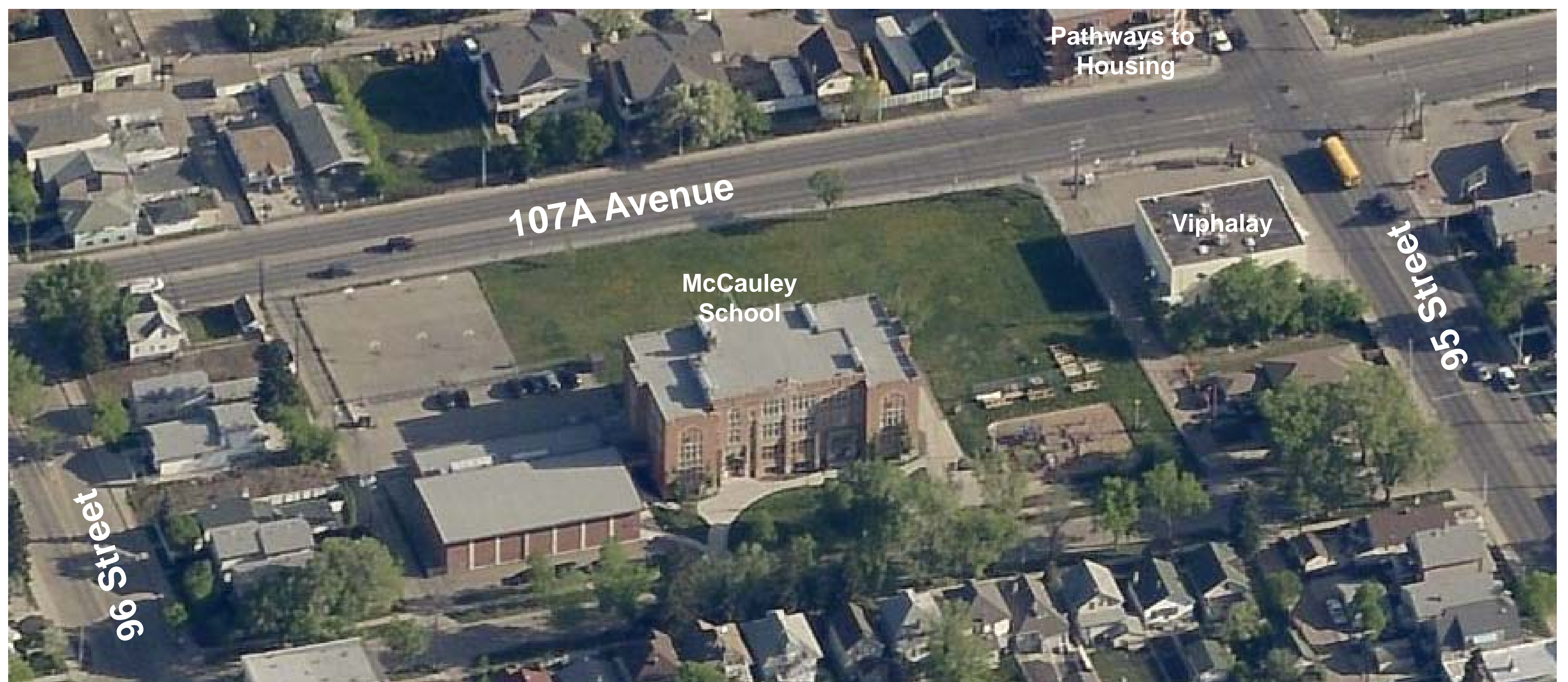
View from South - between 96 Street & 95 Street
