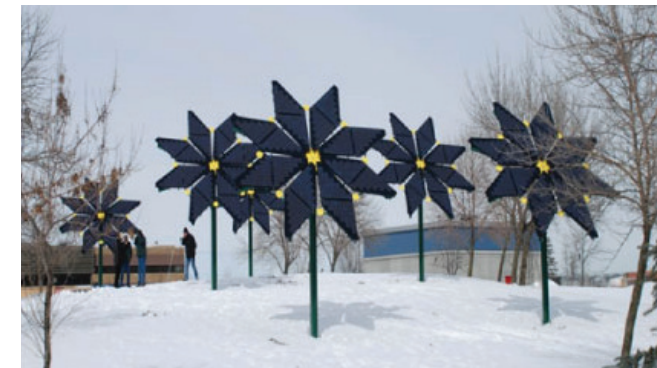
Solar Panels as Public Art Photo Credit: Provident Solar Ltd.
