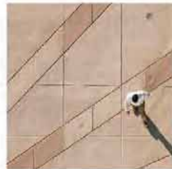
Paving (Patterned Concrete)
