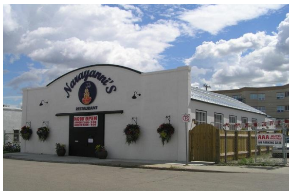
Arndt's Machine Shop before and after restoration
