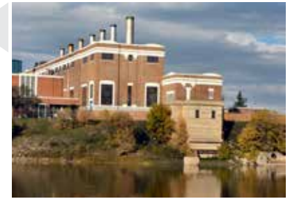
Rossdale Power Plant
